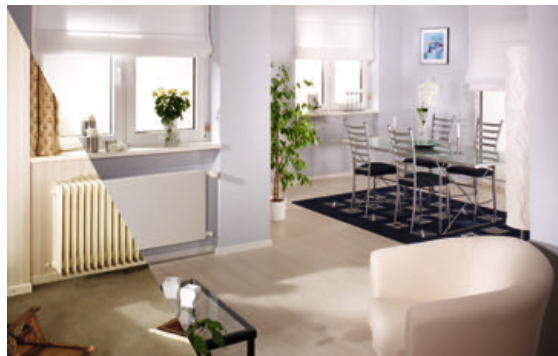
Fig. 70: Fitting accuracy at the time of modernisation of the radiators
