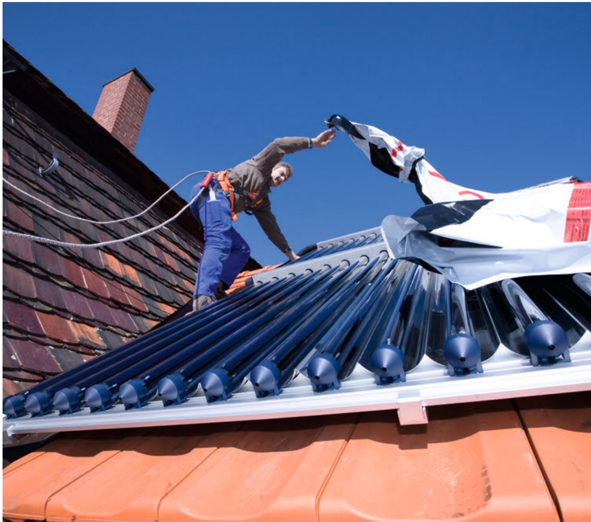
Fig. 53: System example – Vacuum tube collector
